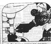
4) The foreign matter has accumulated in the elbow joint, or trap; I take apart the joint.
